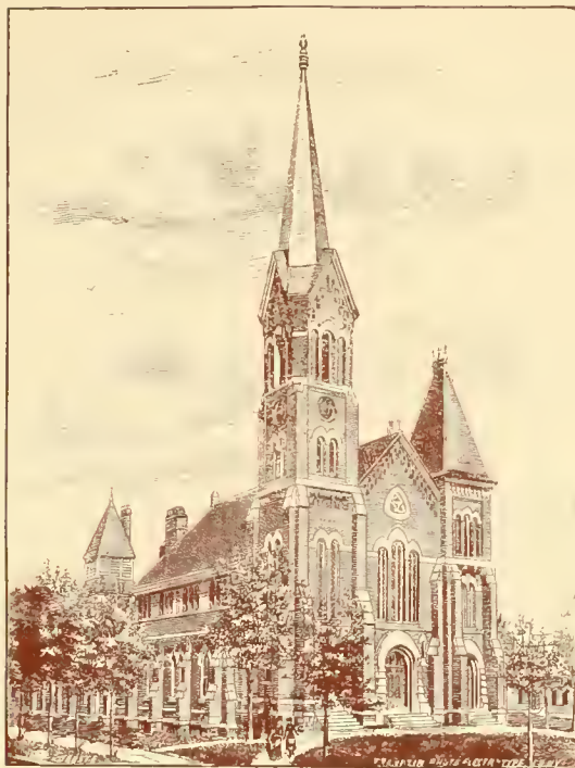
FIRST CONGREGATIONAL CHURCH, FRONT AND MAIN STREETS, BINGHAMTON, N. Y.
